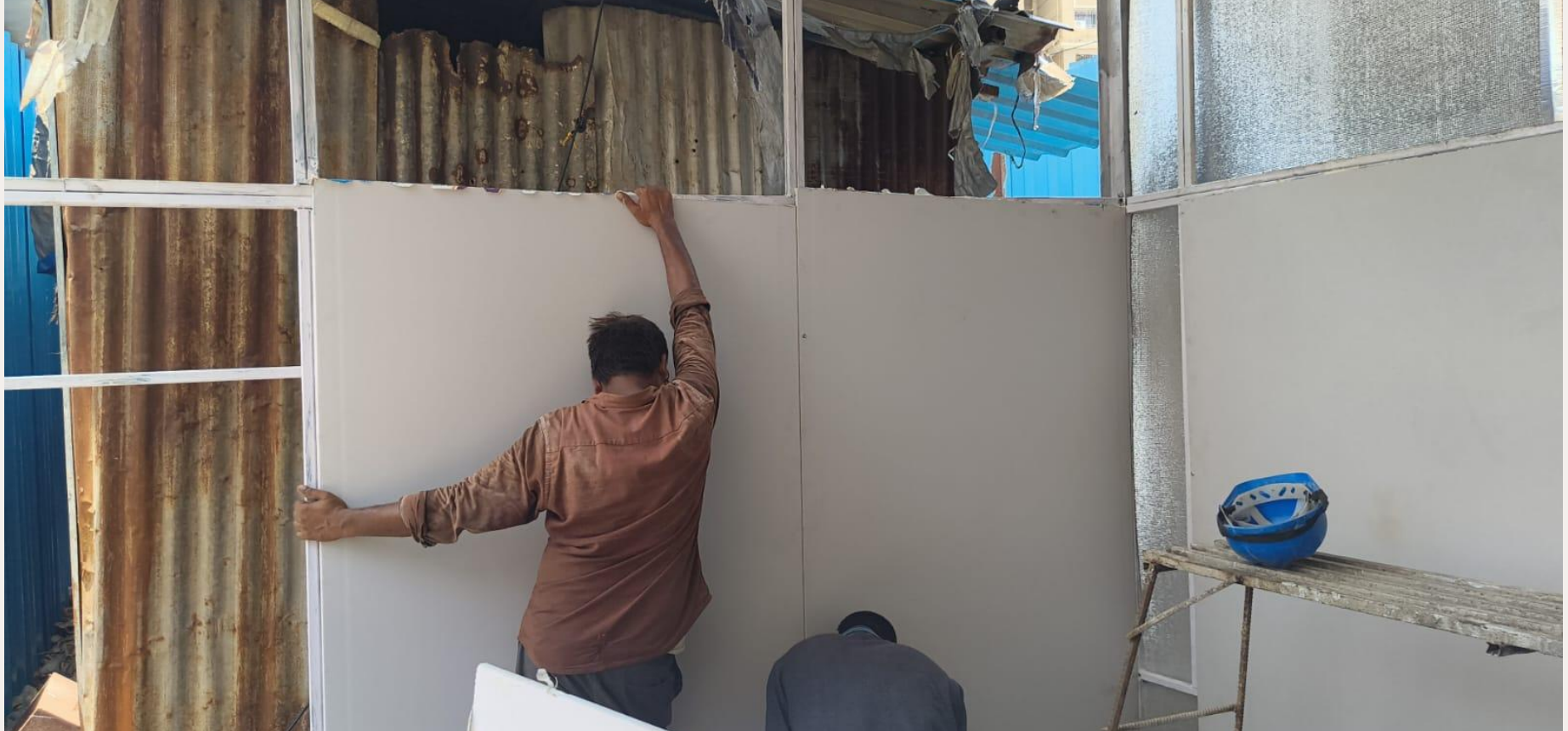
Gyproc (Gypsum) boards being installed to clad the XLPE-Alupet insulation: Thane
