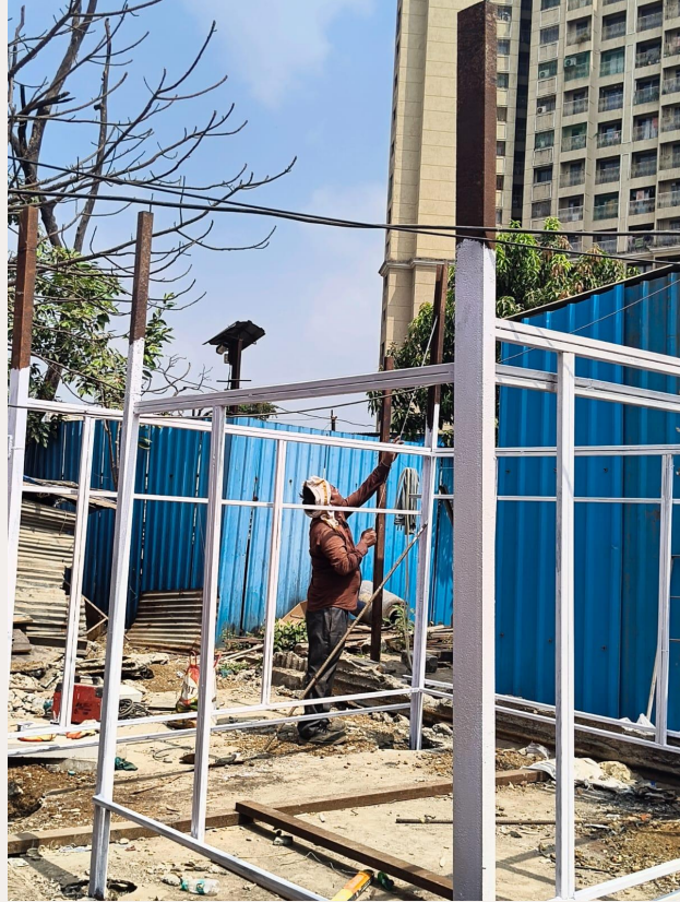
Left, preparation of the frame structure for the composite walling, Right, application of the anti rust paint, cladding sheets Thane
