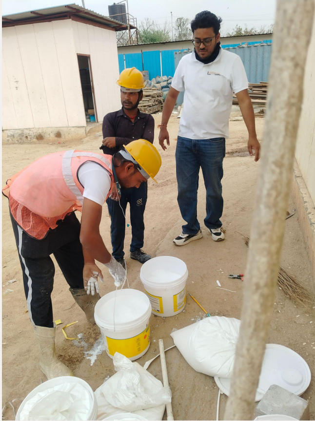
Left: Preparation, and mixing of the high SRI Paint (Luminx), Right: Application of the high SRI paint on the PPGI roofing units Gurgaon
