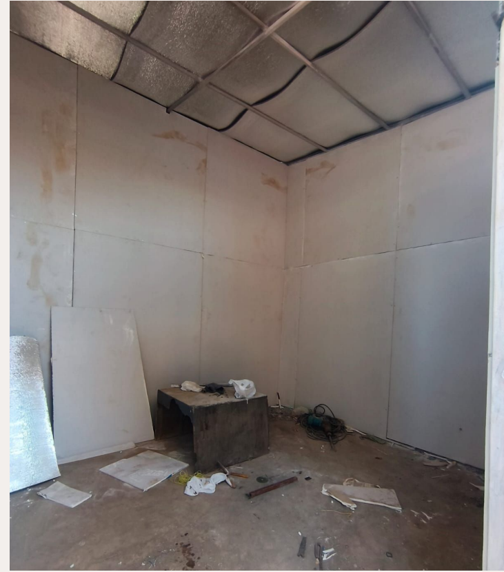
Left: Cluster of 3 demonstration units, complete with overhead clerestory windows for passive ventilation, Right: internal cladding; Gyproc boards - Alupet Foam - PPGI sheets
