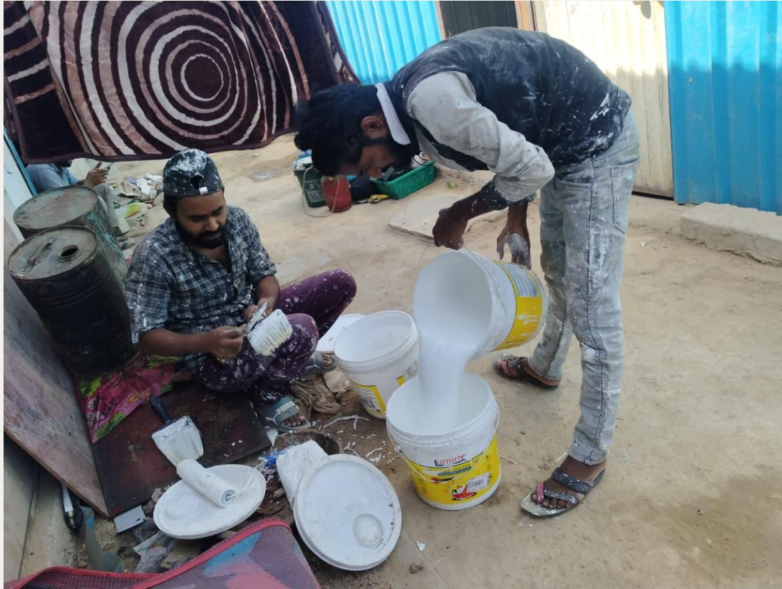
Site workers preparing and applying the High SRI paint manually following a workshop, Gurgaon
