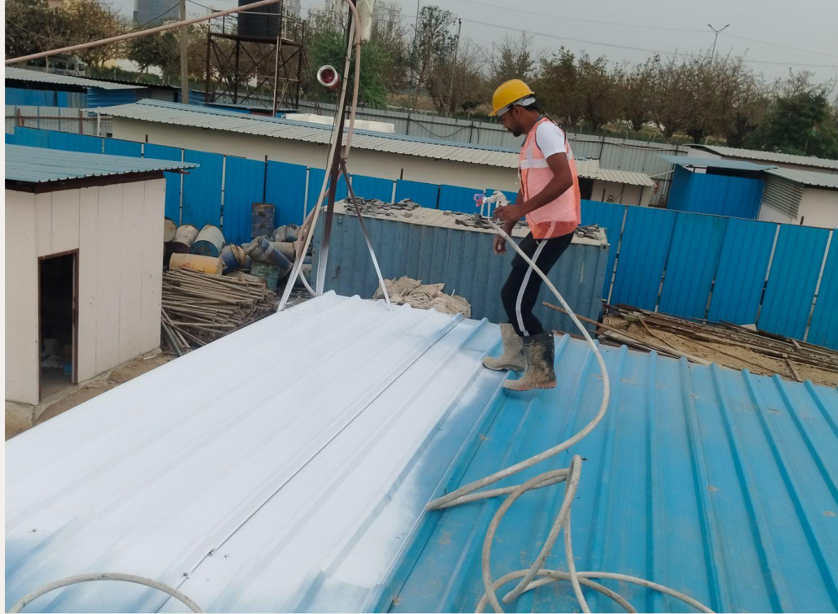
Left: Preparation, and mixing of the high SRI Paint (Luminx), Right: Application of the high SRI paint on the PPGI roofing units Gurgaon
