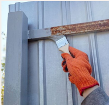
J. Anti Rust Protective Paint on Metal Structural Sections
