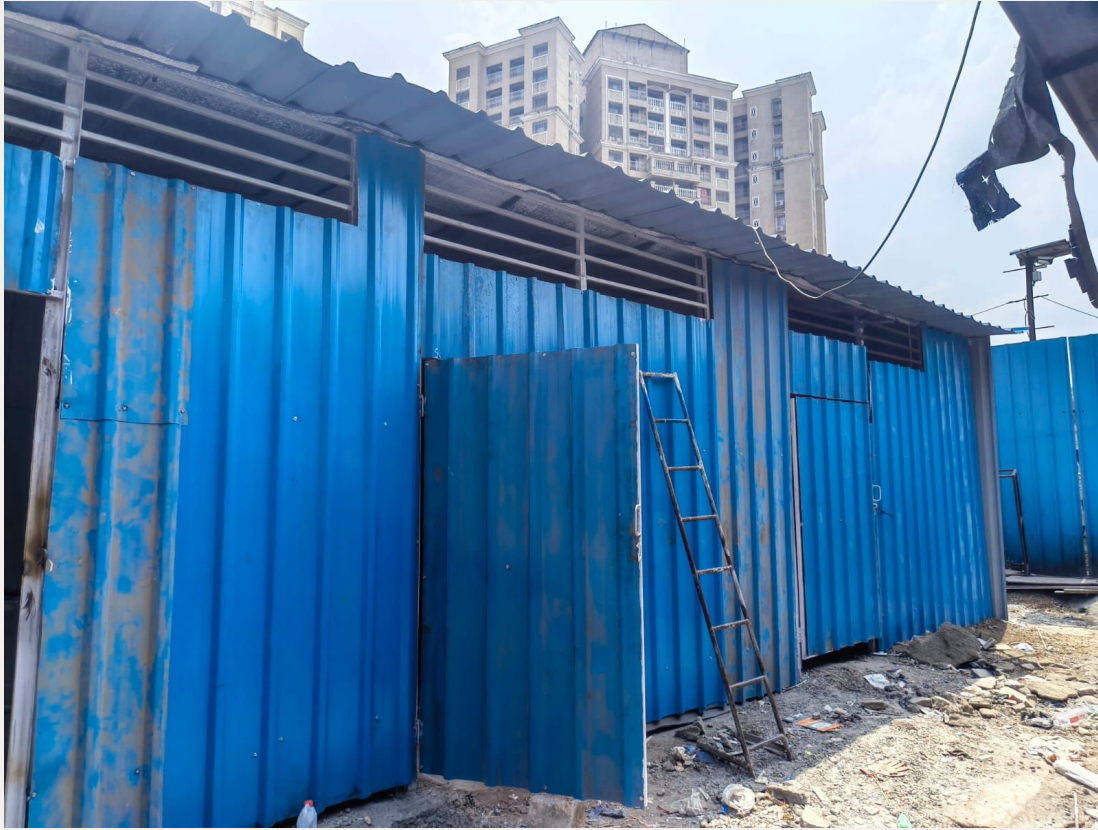
Left: Cluster of 3 demonstration units, complete with overhead clerestory windows for passive ventilation, Right: internal cladding; Gyproc boards - Alupet Foam - PPGI sheets
