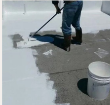
C. Solar Reflective Paint (Luminx) for Walls and Roof
