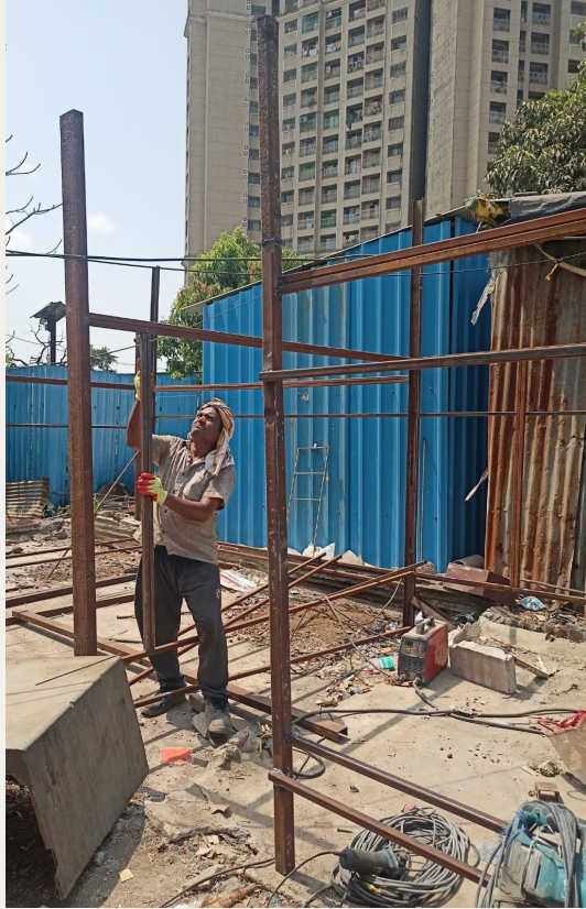
Left, preparation of the frame structure for the composite walling, Right, application of the anti rust paint, cladding sheets Thane
