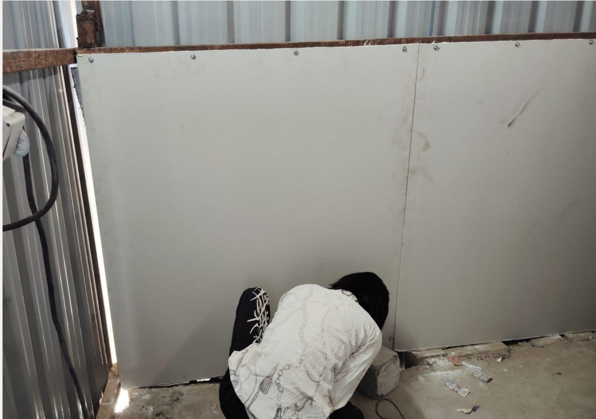
Replacement of Tin sheets with pre-painted galvanised iron sheets (PPGI), insulation and internal cladding: Gurgaon
